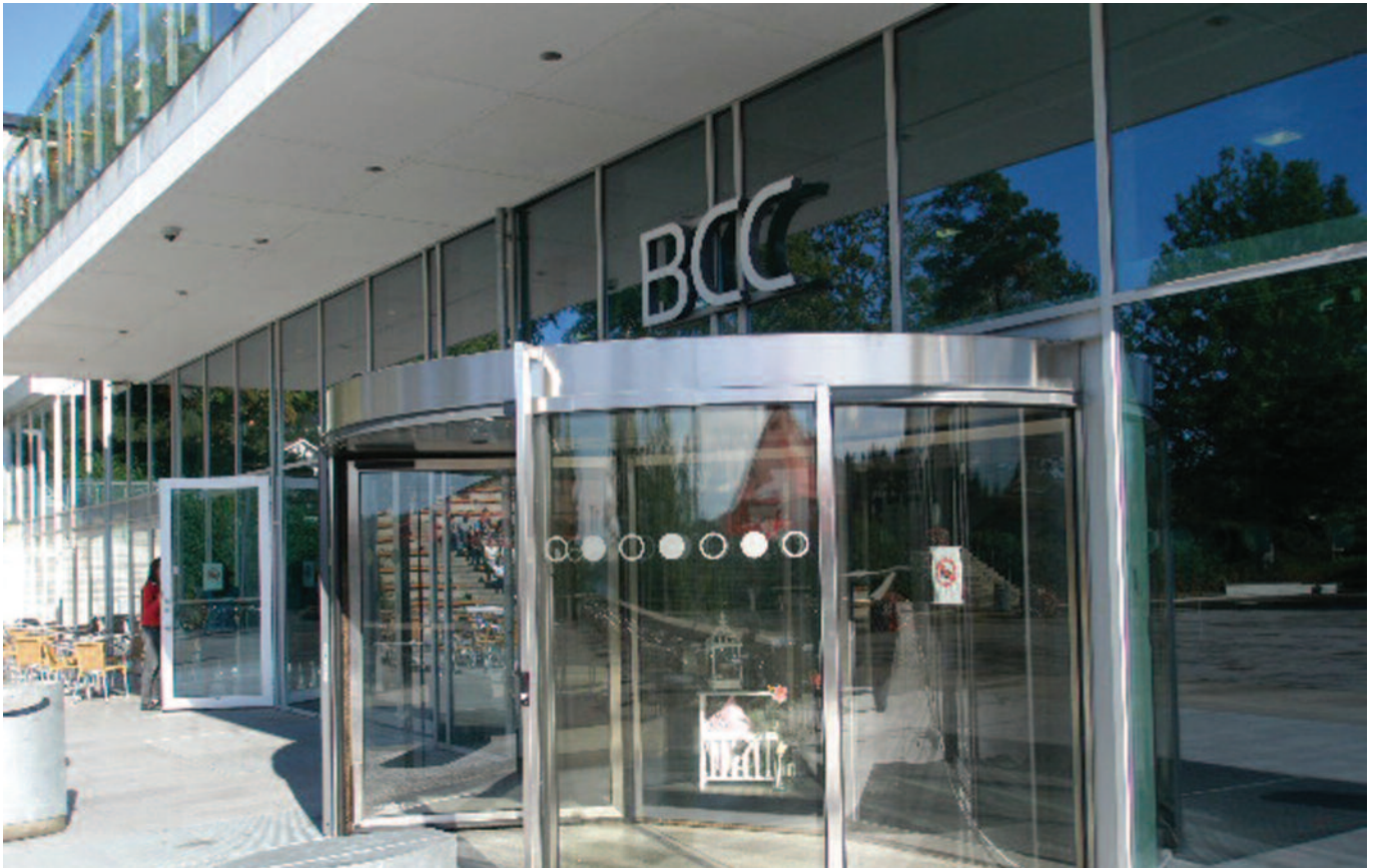
Fig. 1. A revolving door made from stainless steel that appears free from rust at first sight.
